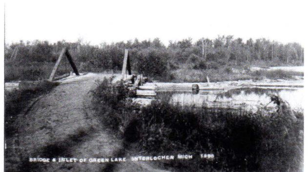
Bridge over the Little Betsie 1908 approximately 100 feet from the mouth of the river (the lake shoreline in the distance)
