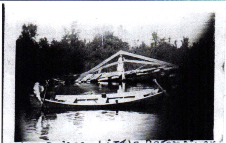
The original Bridge over the Little Betsie
